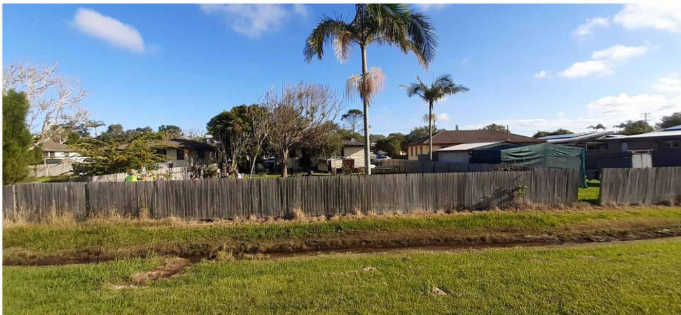
PHOTO 05 - 44-46 EIGHTEENTH AVENUE FROM PARK
